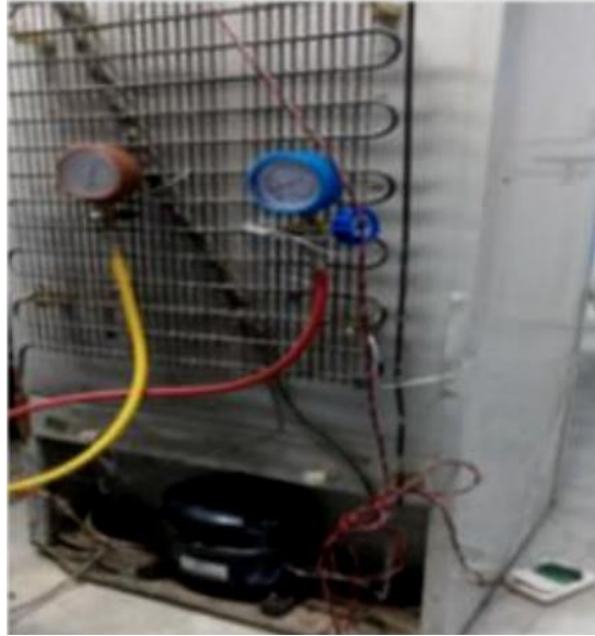
Fig.5: Condenser measuring unit of Refrigerator
